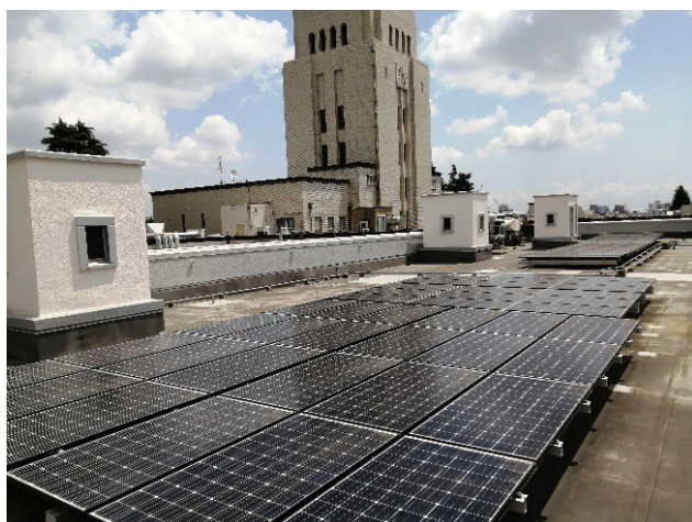
Photovoltaic power generation at the Ookayama Campus main building (10 kW)
